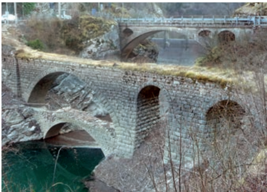
Racli Bridge and the new bridge, in concrete, built after the construction of the dam.
