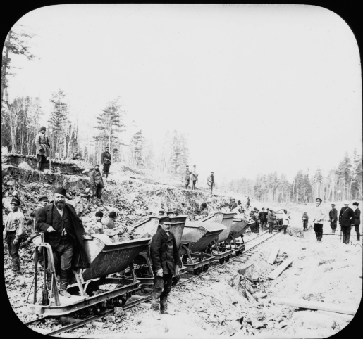
William Jackson, Costruction work on the Eastern Siberia Railway, Khabarovsk 1895 (Cortesia CRAF)
